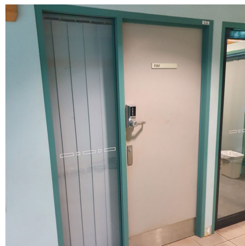
Completed painting works
