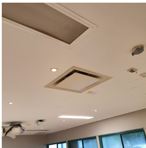
Replacement HVAC unit
