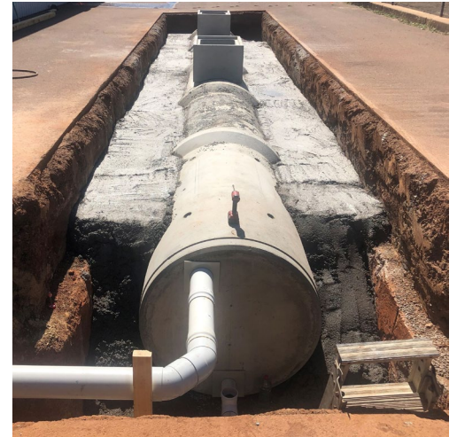
Sewer overflow chamber
