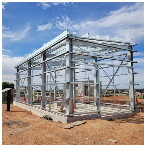
Structural steel construction
