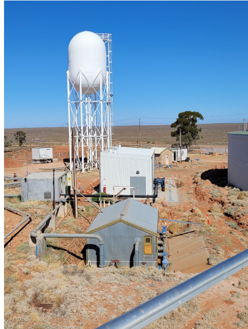
Site overview with newly constructed pump house
