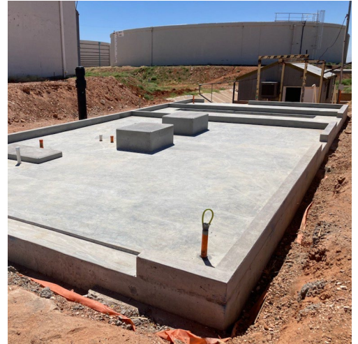
New concrete slab
